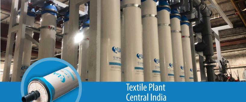
The Q-SEP UF system, designed at high flux rates of 60 LMH, required 30% lesser number of modules to be installed, saving on client's capex.
